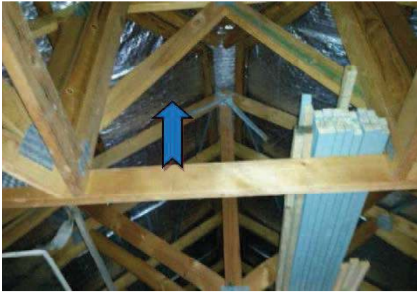
Photo 3. Bldg 242.1, roof lining, sarking insulation suspected to contain SMF.
